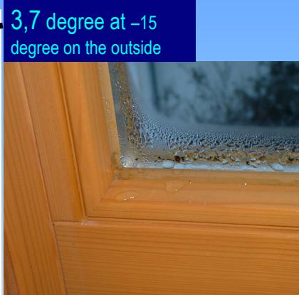
Below an  $U_g$  value of  $1,0 \text{ W/m}^2\text{K}$
