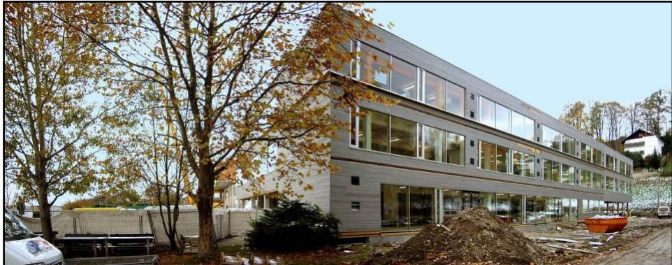
Space heat from 165 kWh/m<sup>2</sup>a to max. 15 kWh/m<sup>2</sup>a
